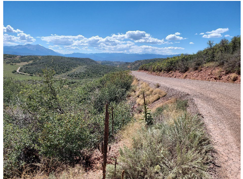
Photo 13. Side slope of the existing roadway
