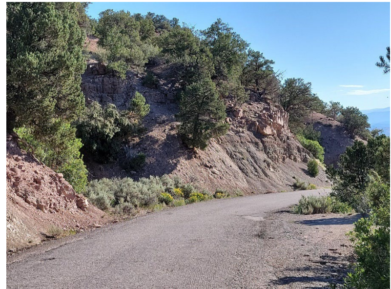
Photo 4. Rock outcrop and weakly cemented surficial soils
