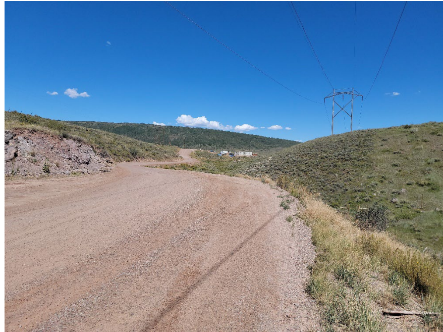
Photo 11. Rock outcrop in the potential cut section
